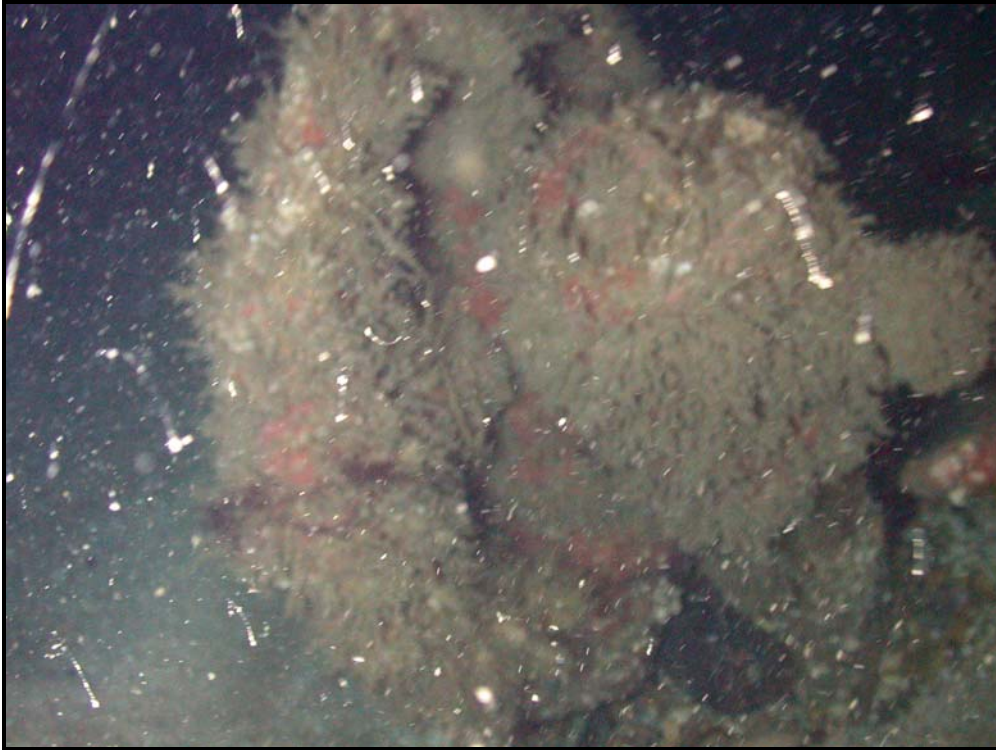
Figure 17. Aft Downton pump.
