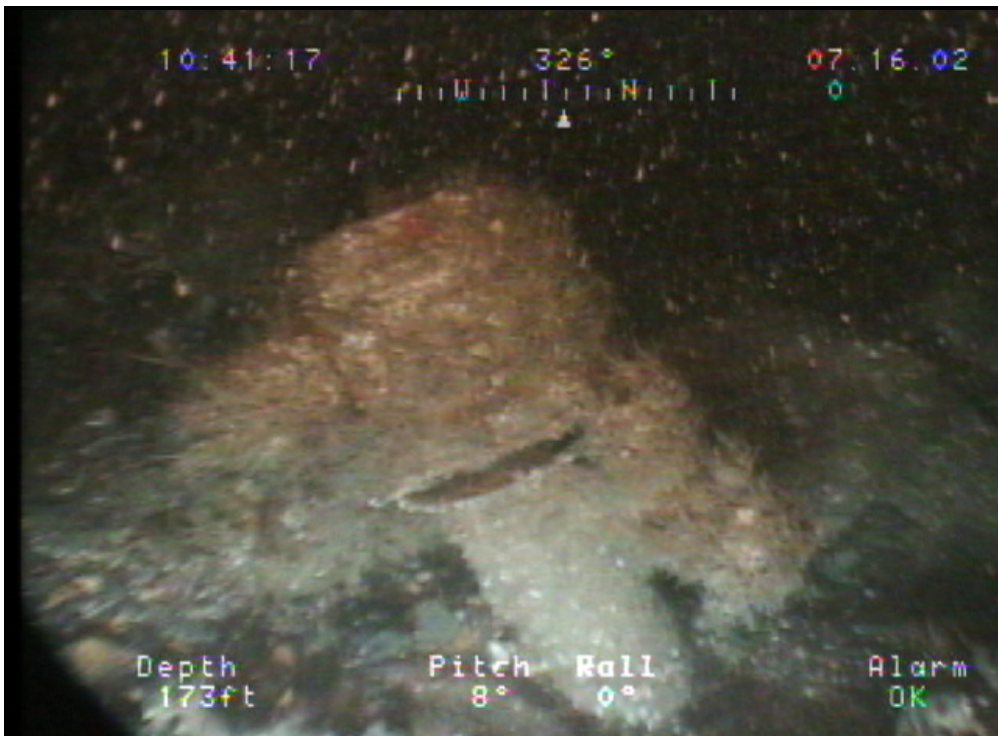
Figure 18. Damaged forward Downton pump.
